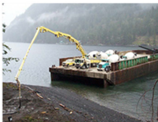
Photo A18: Example of concrete installation by barge
