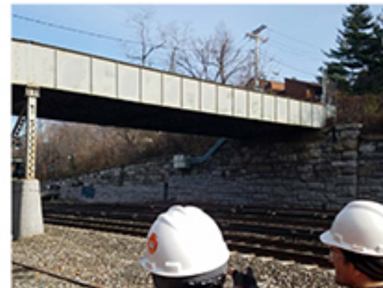
Photo A07: West 254th Street Bridge
