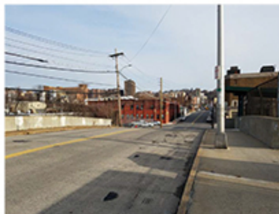
Photo A10: Ludlow Street Bridge over Metro-North tracks, looking east
