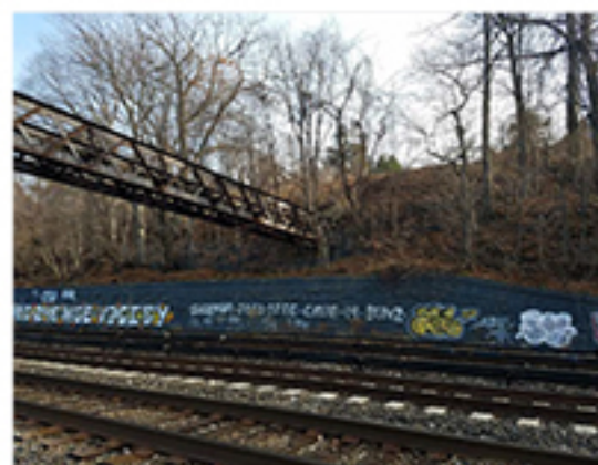
Photo A05: Existing bridge near West 231st Street
