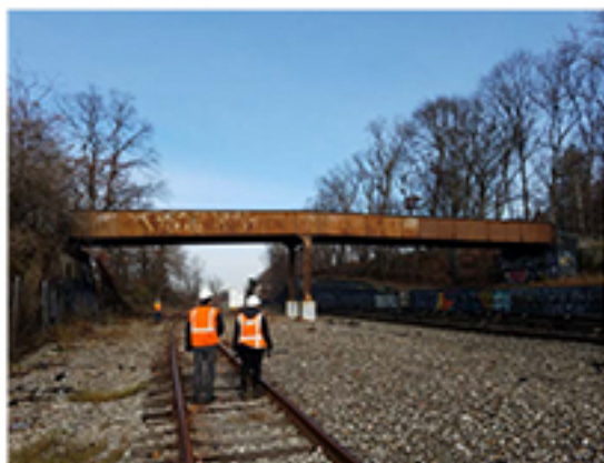
Photo A09: College Point Bridge near West 261st Street
