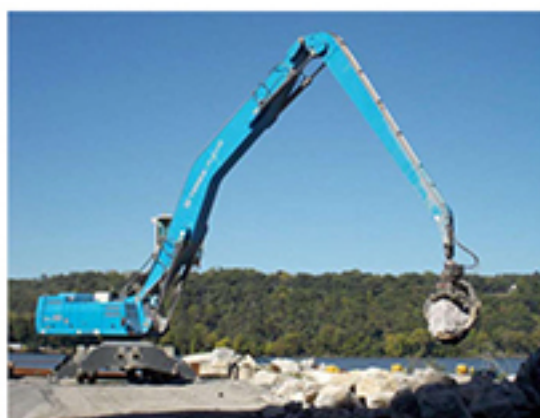
Photo A17: Example of placement of large rip-rap
