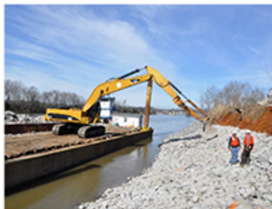
Photo A16: Example of rip-rap installation from a barge
