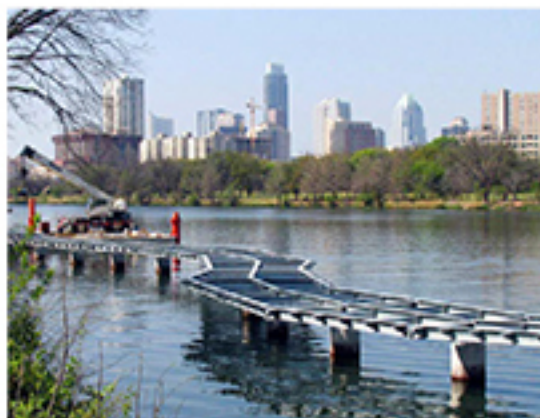
Photo A15: Example of construction of elevated walkway from barge
