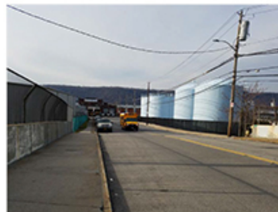
Photo A11: Ludlow Street Bridge over Metro-North tracks, looking west
